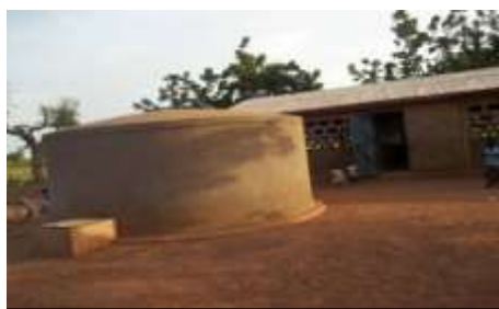
Figure 2: Rainwater Harvesting Tank, Cheshie
