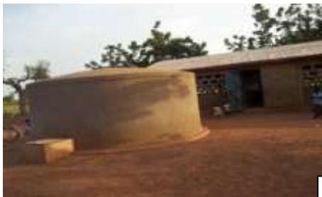
Figure 2: Rainwater Harvesting Tank, Cheshie
